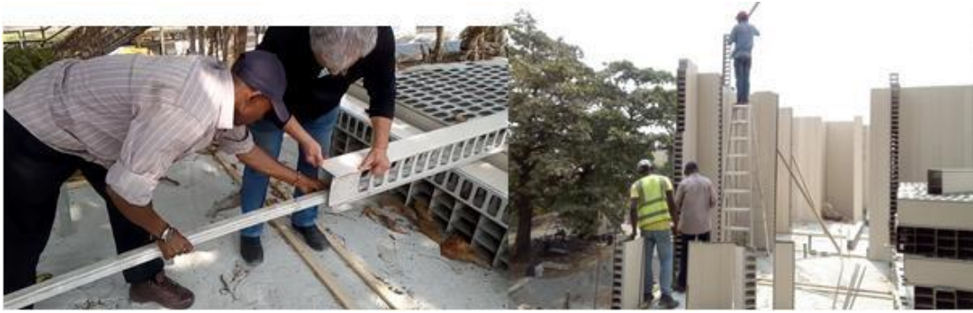
Figure 3. Service duct being inserted on site as worker on the right hammers box and barrel into each other
