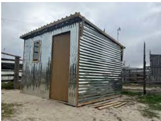
Figure 2: Temporary Shack structure
