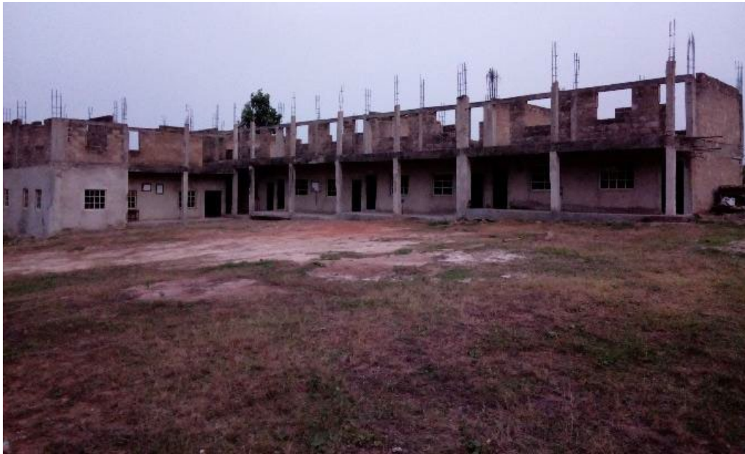
Figure 1: The building under evaluation
